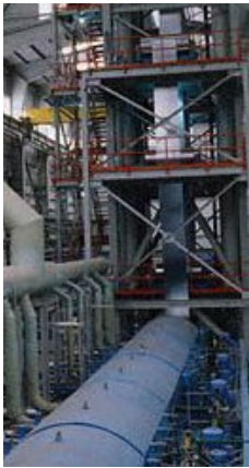
SAFE LUBE™ products may be used in steel manufacturing
